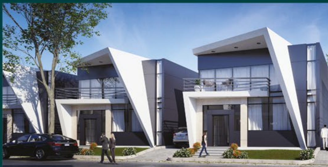
Live view Villas Villas residential compound at Al Shorouk City
